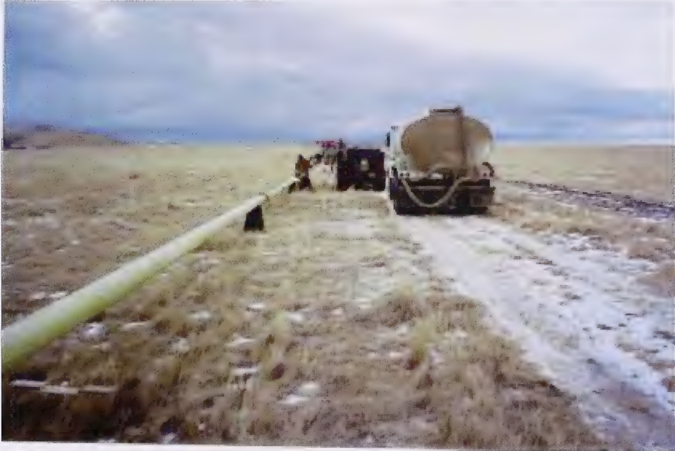
Photo 23 Wild fire control is an important issue to ranchers during periods of drought. In this photo a water truck accompanies the welding crew.
